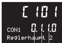
Main controller configuration 2:
